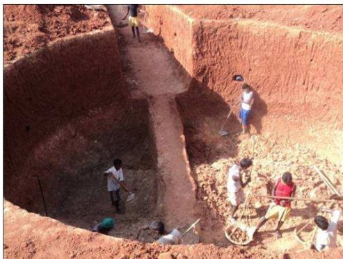
Construction of an irrigation well, Rokedega
